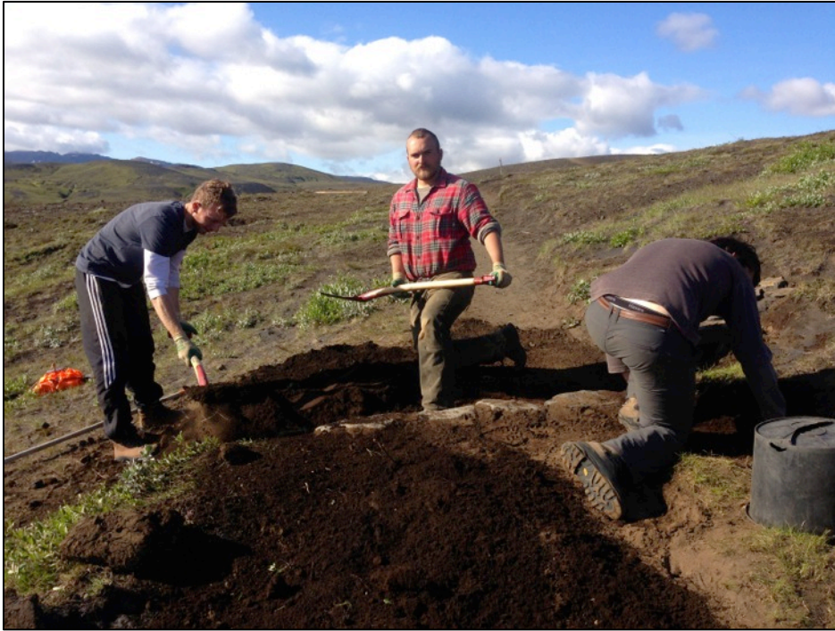
Stone water bar construction
