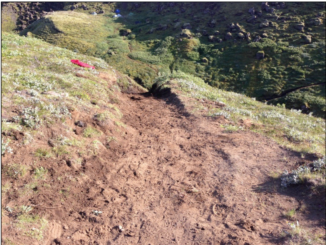
(Before and After) Reprofiling and filling the gullied trail. Stone waterbars were constructed upslope to prevent further damage from water.
