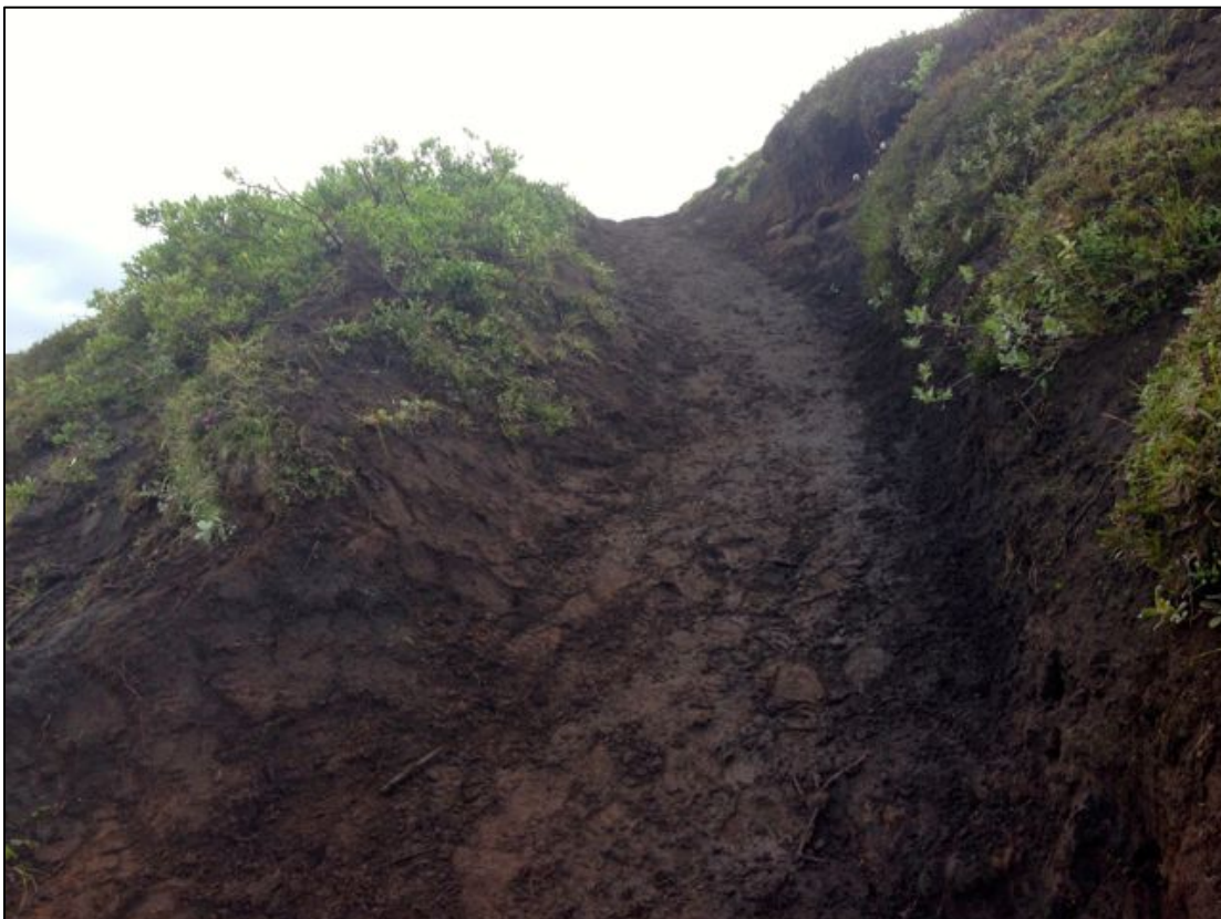
(Before and after) Undercutting and reprofiling of the slope. Remaining vegetation is replanted to cover exposed roots and establish a growing surface. A small amount of fertilizer is added to promote regrowth.
