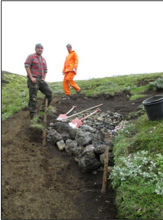
(During) Stone added to eroded area.
