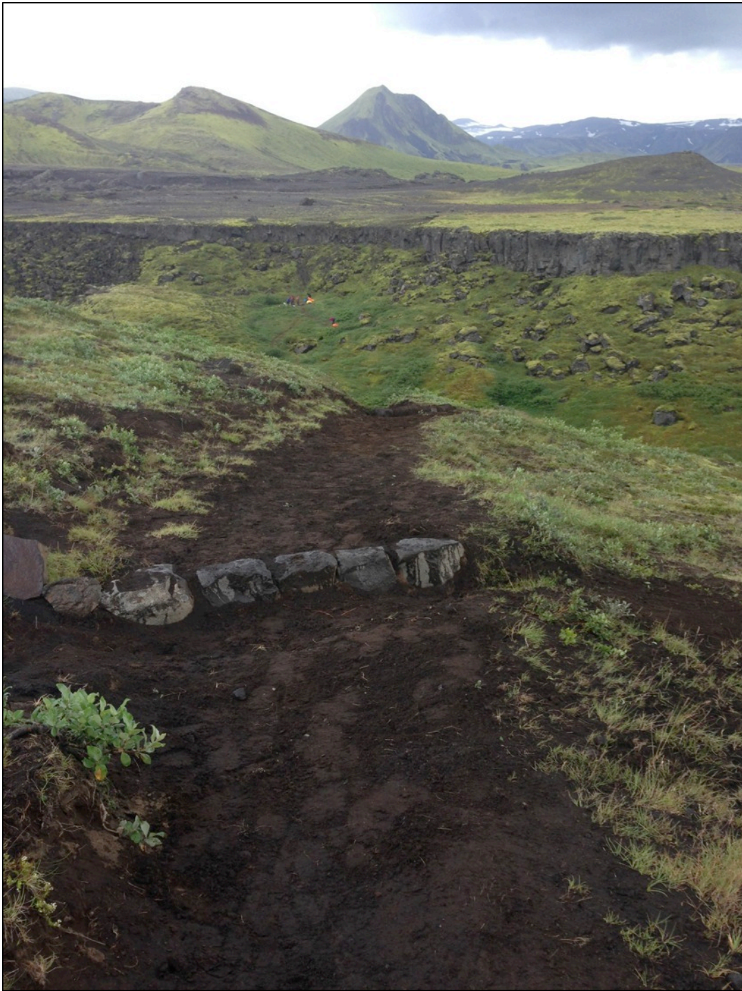
(After) Stone waterbar build to protect the repaired trail and slope ahead. The left side of the trail has been regarded where the bank has been undercut and filled. Turf has then been replanted.
